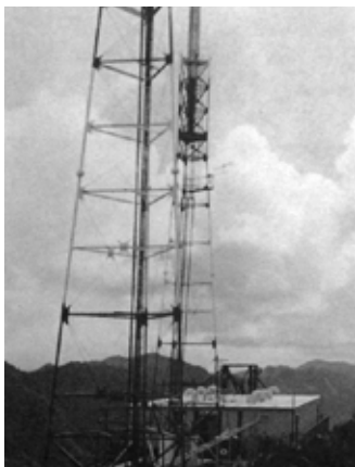
NEWLY BUILT TRANSMISSION TOWERS
