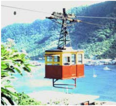
ORIGINAL AERIAL TRAMWAY USED FOR CONSTRUCTION AND TOURISM
