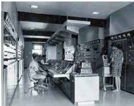
TRANSMITTER CONTROL AT TOP OF MT ALAVA
